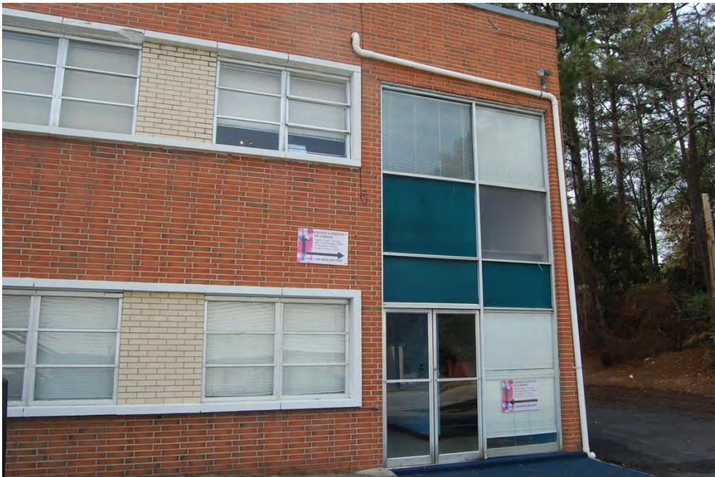
Plate 9. Stewart Building, Windows and Rear Entrance, Looking West.
