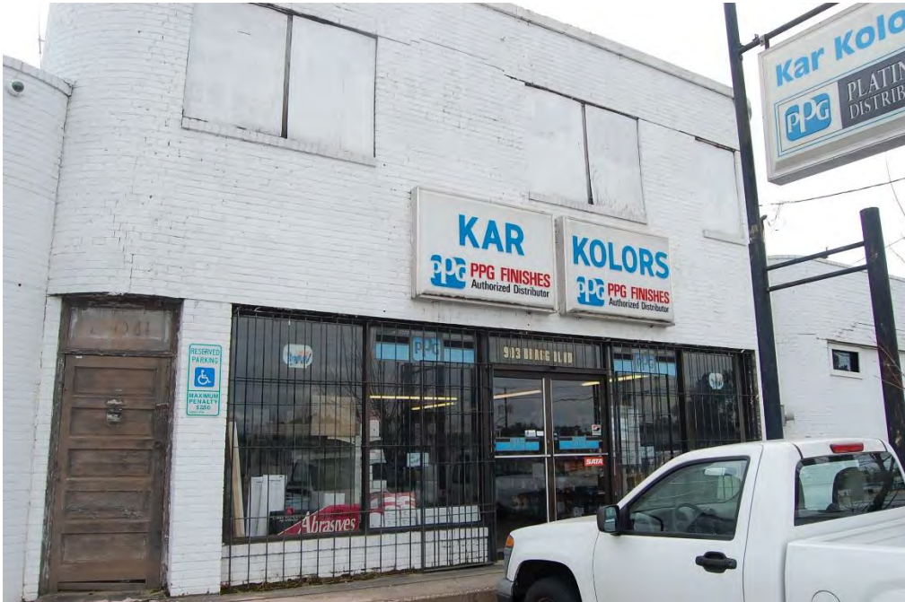
Plate 27. Moore's Market, Façade, Center Block, Looking South.
