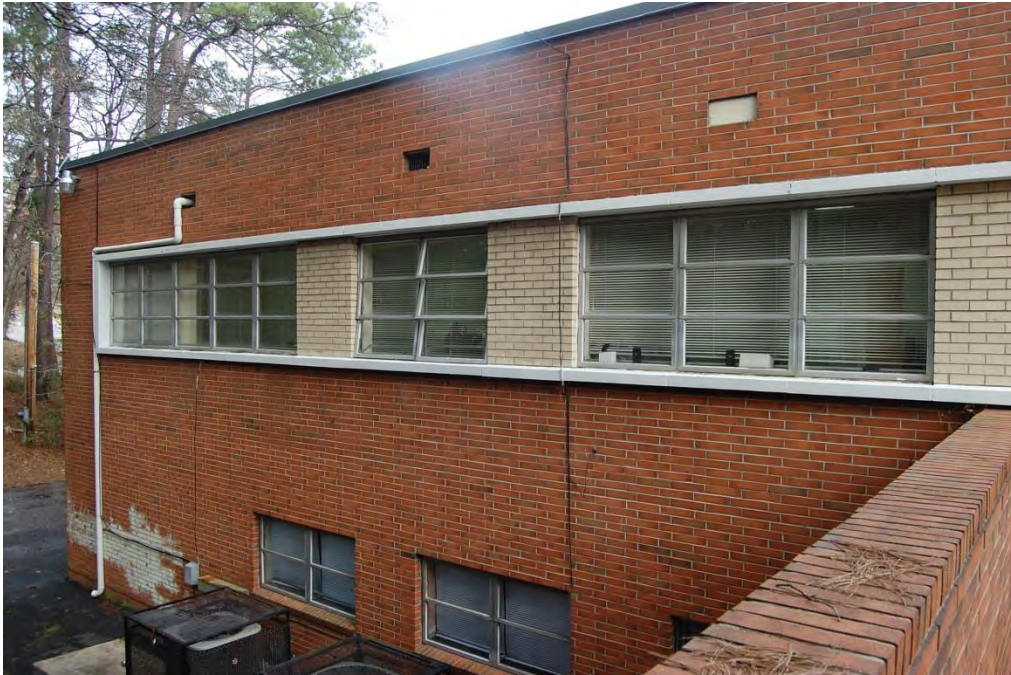
Plate 6. Stewart Building, Side (West) Elevation, Looking Northeast.
