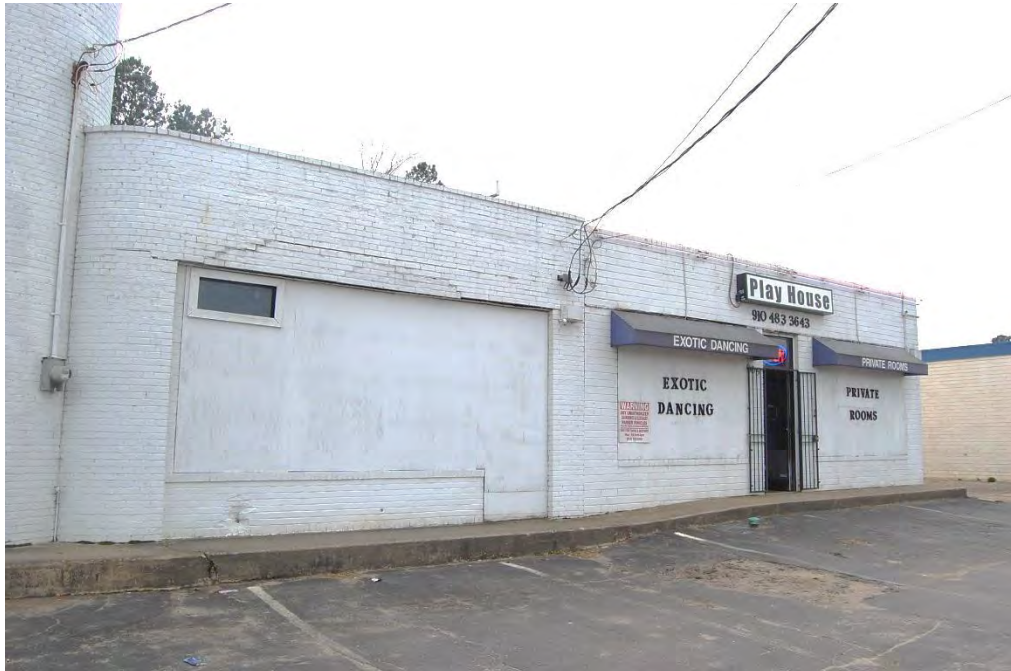
Plate 29. Moore's Market, West Wing and 1960 Storefront Addition, Looking South.
