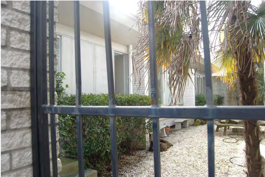
Plate 48. Dr. Robert Lessom Dental Office Building, Side (West) Elevation, Looking South.
