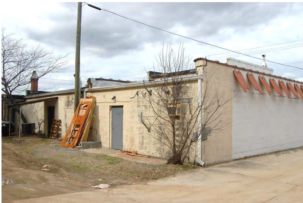
Plate 32. Moore's Market, Rear Elevation, Looking North.
