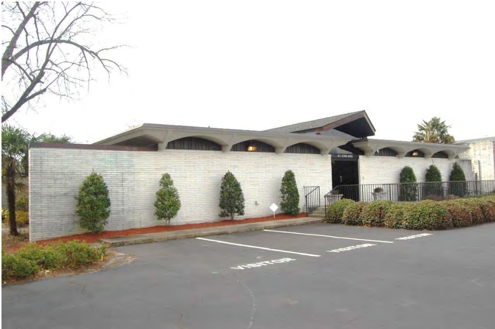
Plate 45. Dr. Robert Lessom Dental Office Building, Rear (North) Elevation, Looking Southwest.
