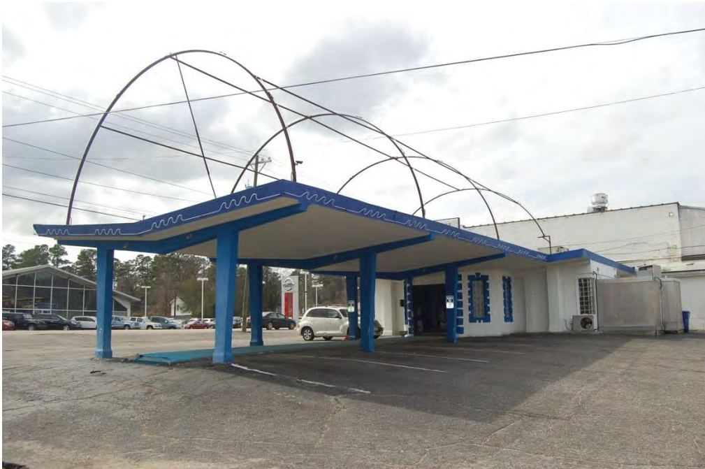
Plate 39. A&W Drive-In Restaurant, Rear (North) Elevation and Canopy, Looking Southwest.
