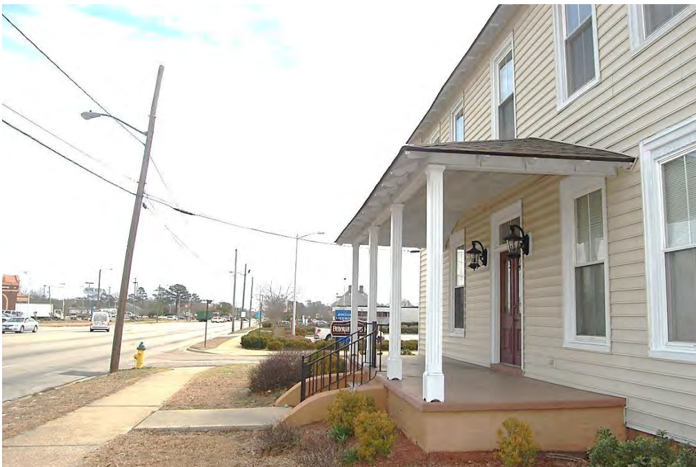
Plate 54. Fennell-Strange House, House and Setting, Looking East Along Rowan Street.
