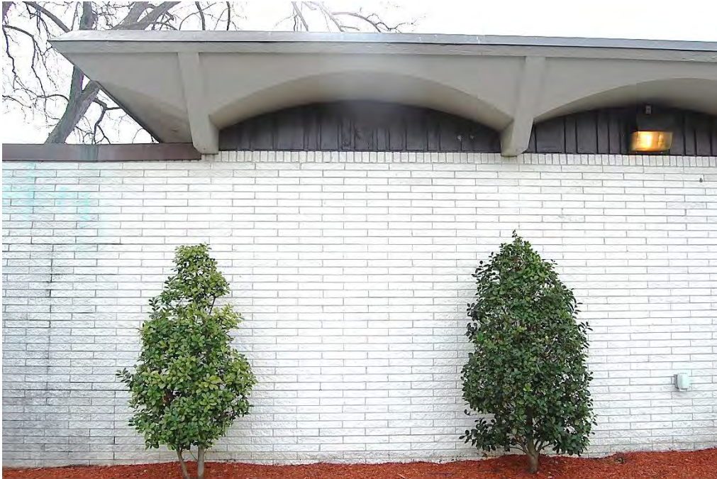
Plate 46. Dr. Robert Lessom Dental Office Building, Rear Elevation, Looking South.
