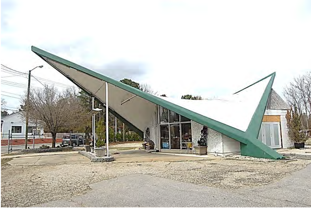
Plate 33. Pam-Oil Gas Station, Looking Northeast.
