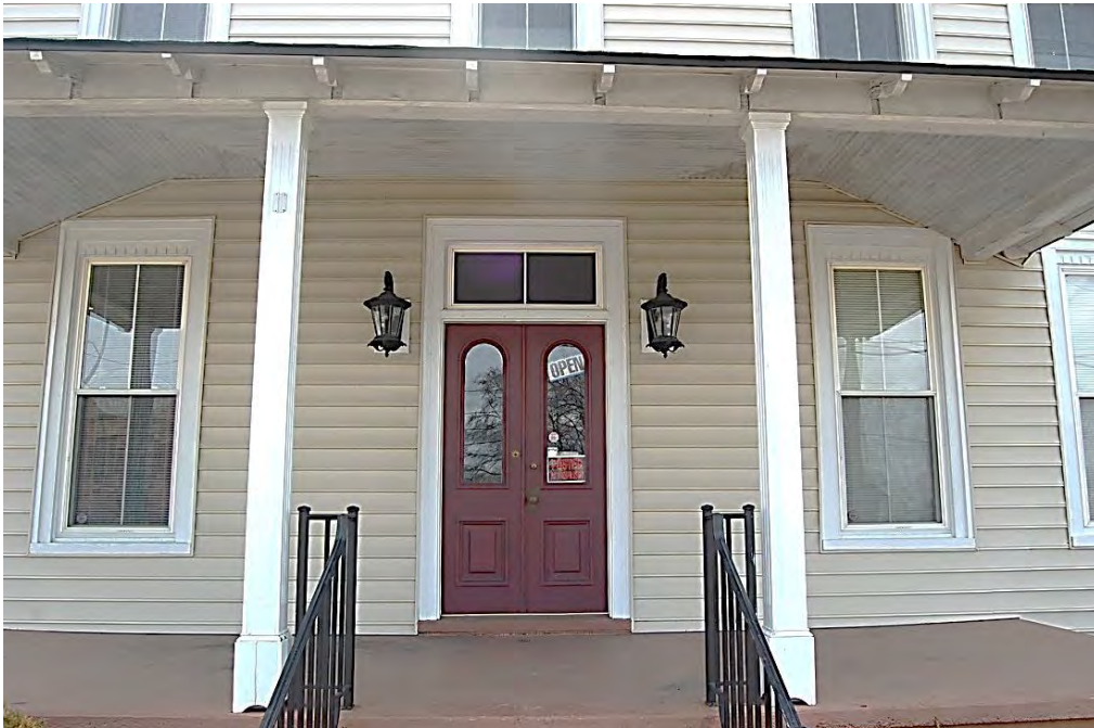
Plate 56. Fennell-Strange House, Façade, Entrance Detail, Looking South.
