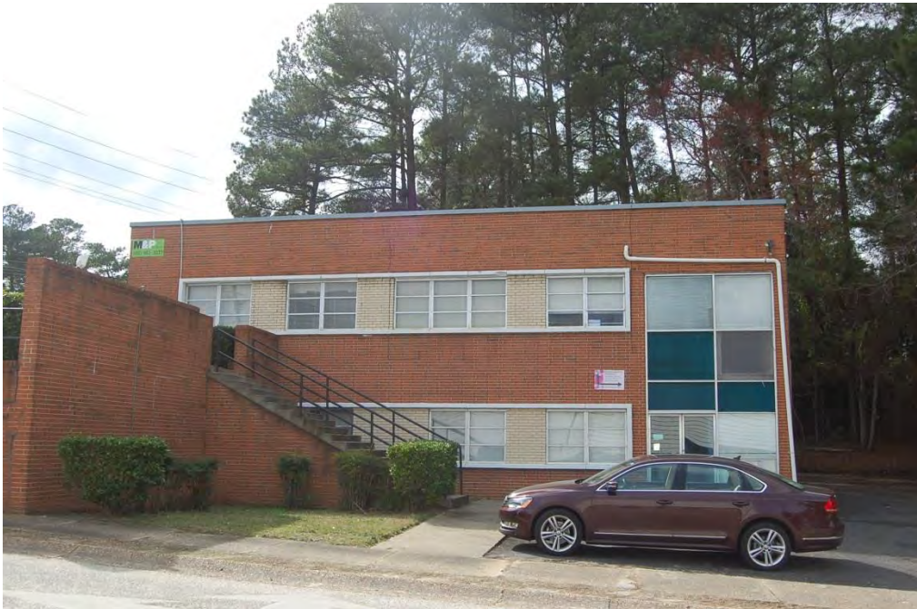
Plate 5. Stewart Building, Side (East) Elevation, Looking West.
