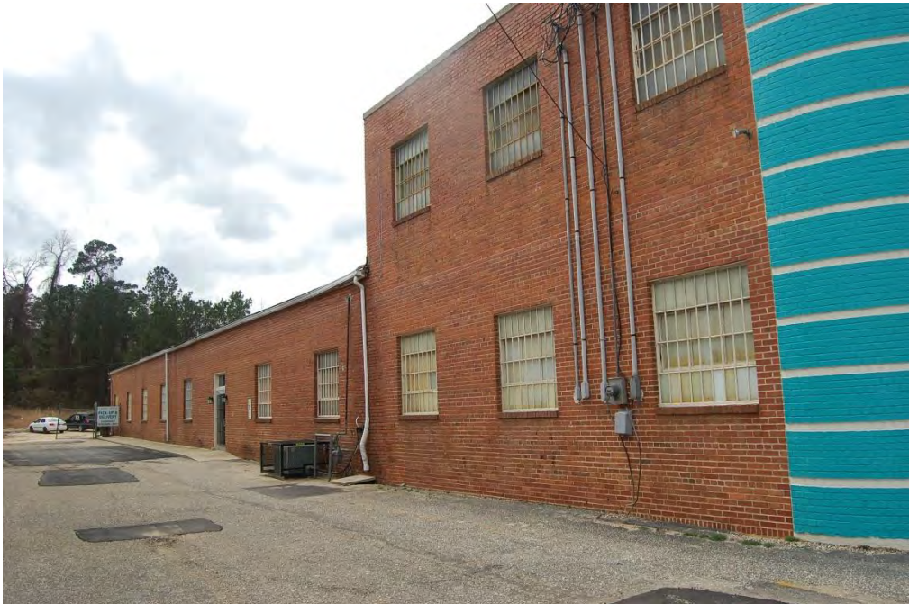
Plate 22. Canada Dry Bottling Company Building, Side (East) Elevation, Looking South.
