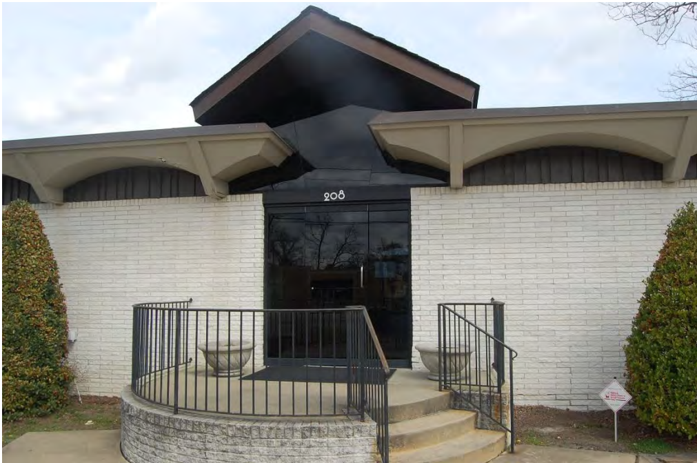
Plate 43. Dr. Robert Lessom Dental Office Building, Front Entrance Bay, Looking North.
