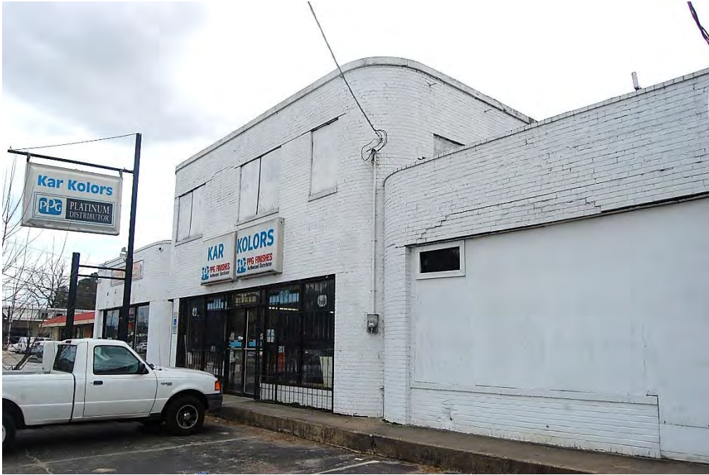
Plate 26. Moore's Market, Façade, Looking Southeast.
