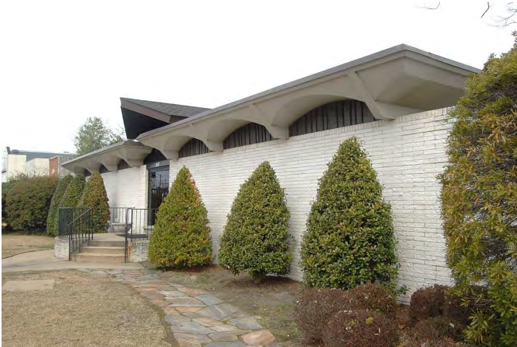
Plate 44. Dr. Robert Lessom Dental Office Building, Facade, Looking Northwest.
